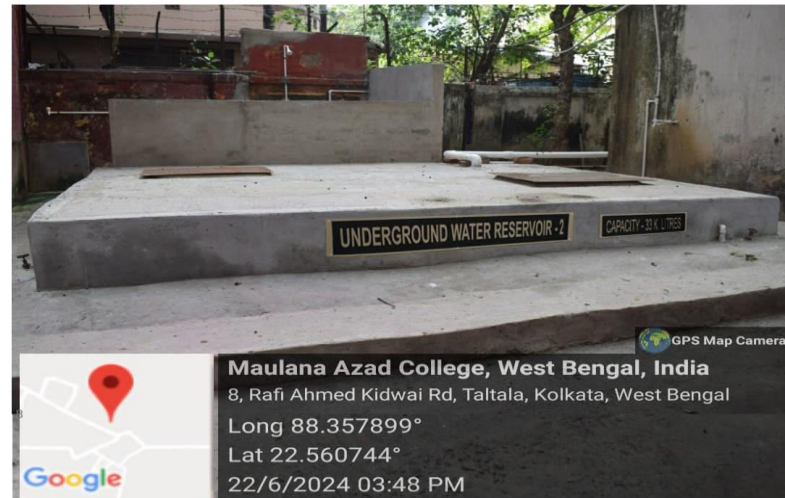
Underground water reservoir 1 (40K lts. Capacity) Underground water reservoir 2 (33K lts. Capacity)
