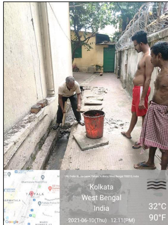
Drain clearance and maintenance within College campus
