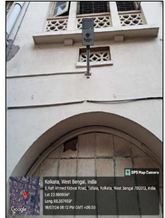
SOLAR PANEL AT THE COLLEGE ROOFTOP (LEFT) AND THE SOLAR SENSOR BASED COMPOUND LIGHT LINKED WITH IT (RIGHT)
