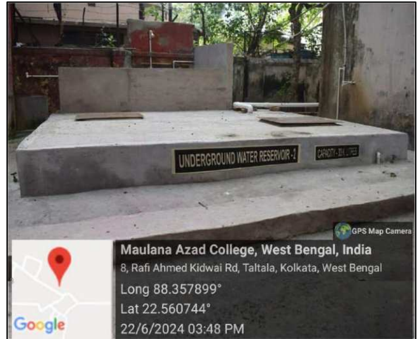
UNDERGROUND WATER RESERVOIR 2 (33K LTS. CAPACITY)
