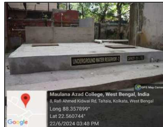
UNDERGROUND WATER RESERVOIR 2 (33K LTS. CAPACITY)
