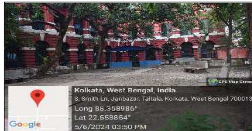
BUILDING OF BAKER GOVT. HOSTEL
