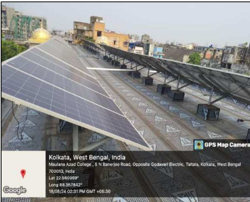
INSTALLED SOLAR PANEL ON COLLEGE ROOFTOP
