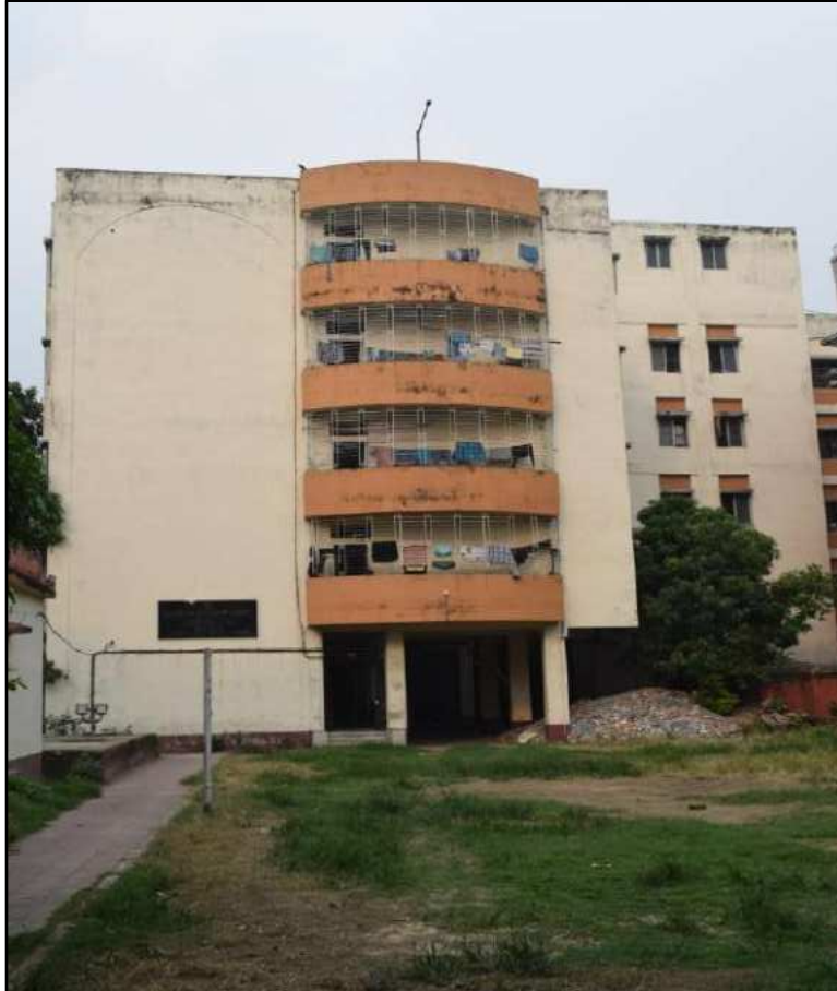
ANNEX BUILDING OF BOYS' HOSTEL
