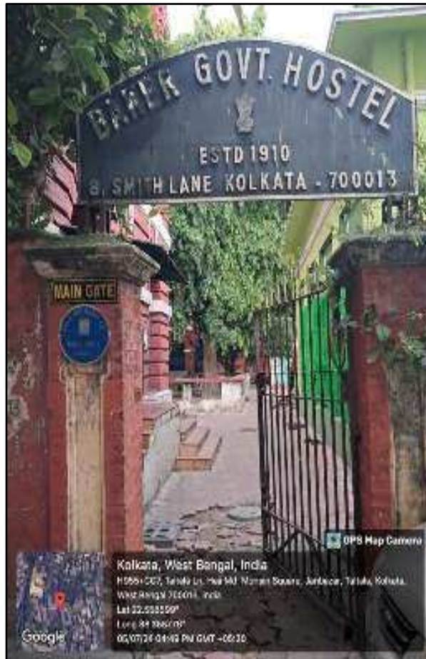
ENTRANCE OF BAKER GOVT. HOSTEL
