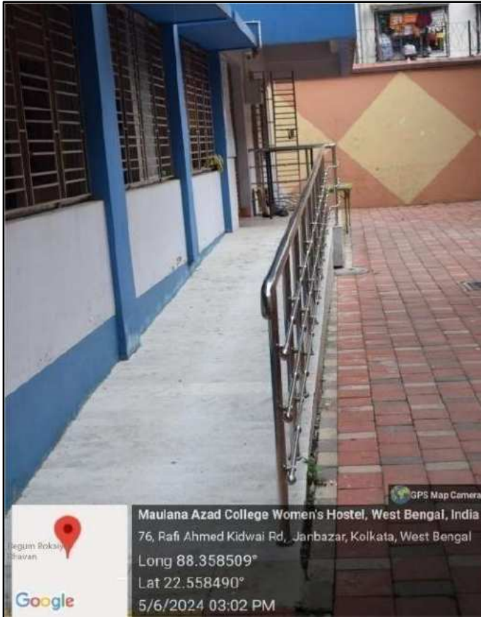
RAMP AND RAIL FOR DIVYANGJAN INMATES
