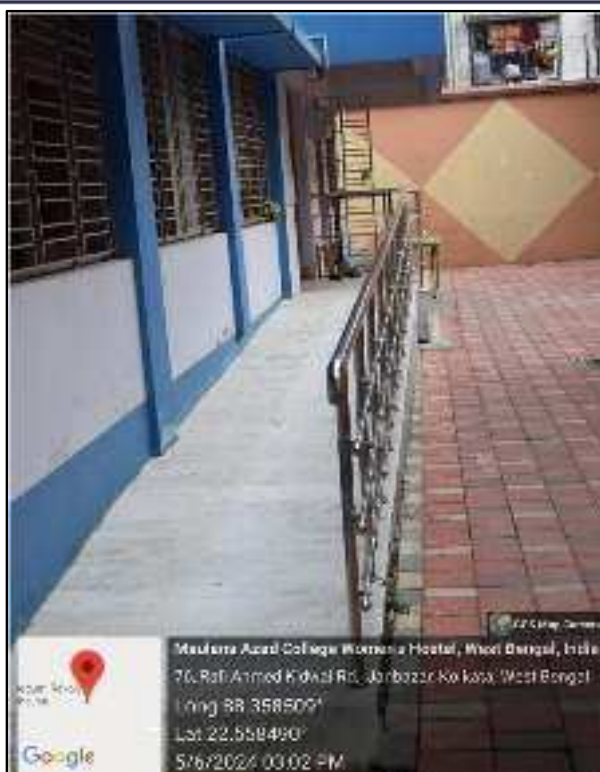
RAMP AND RAIL FOR DIVYANGJAN INMATES
