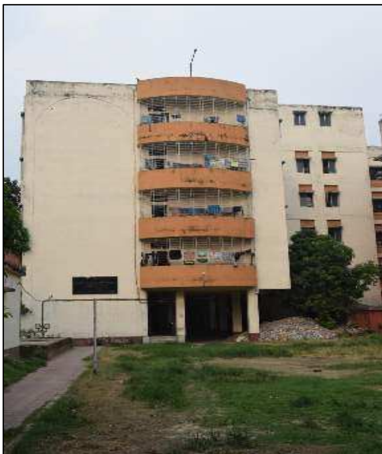
ANNEX BUILDING OF BOYS' HOSTEL
