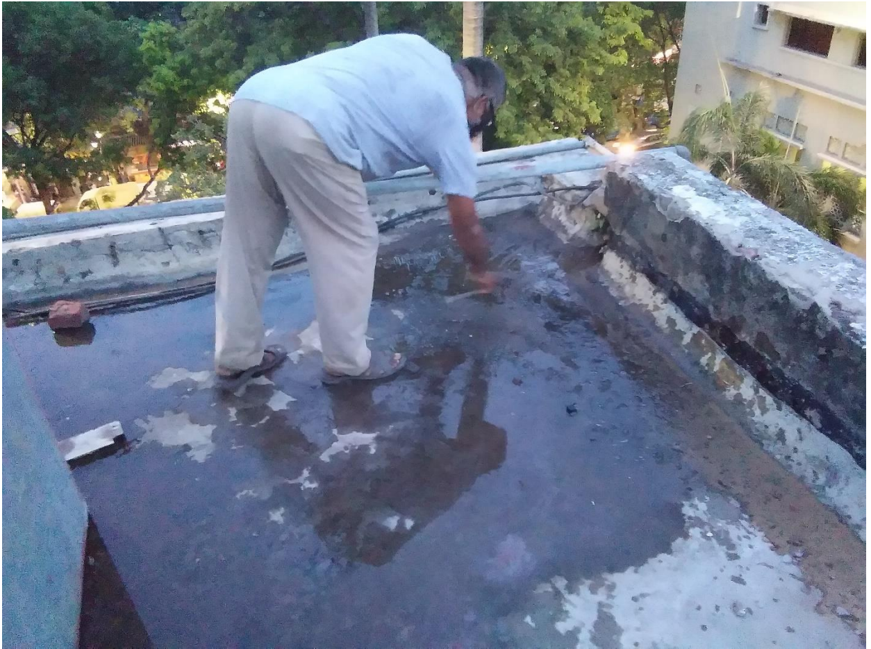
[Roof-top rain water clearance by Staff on 7 th July, 2020]
